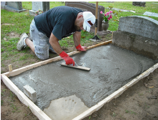
Troweling the concrete
