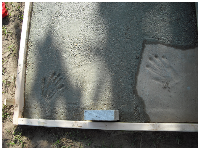
Troweling the concrete
