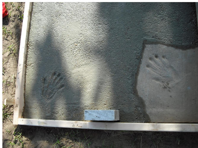
Troweling the concrete
