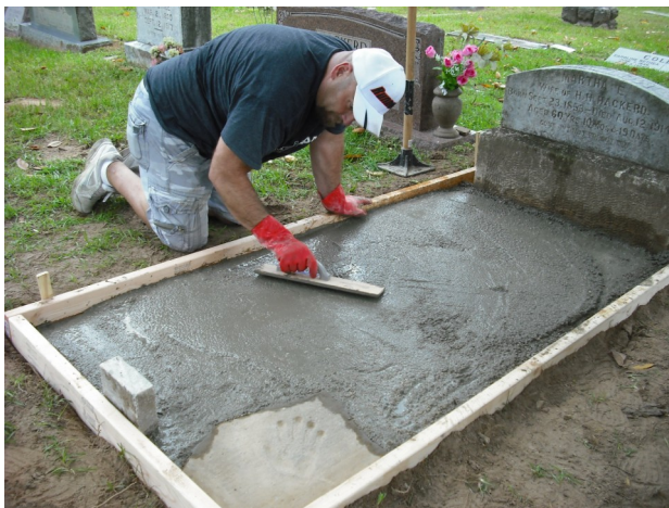
Troweling the concrete
