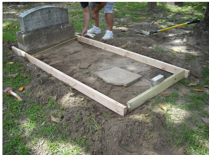
Measuring the framing the new concrete slab
